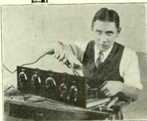
Front View KD-50 Neutrodyne Being Assembled
